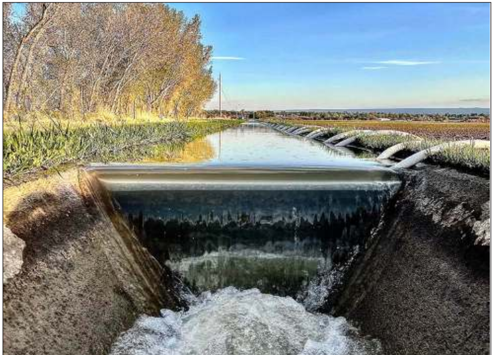
▲ Colorado’s water for agriculture is fed by four major river systems that are connected to the more than 4,000 lakes and reservoirs: The Platte River (northern Front Range); the Arkansas River (southern Front Range); the Rio Grande River (southern); and the Colorado River (Western Slope). A water system in Delta County is pictured. Source: Colorado Department of Agriculture
